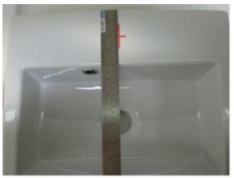
On the upper level of the tap mark the centre of the hole from the rear of wash-hand basin as taken from the measurement on the technical specification.
